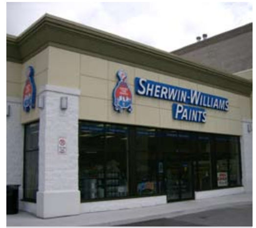
Westney Mall Ajax, Ontario LEED-Certified candidate
