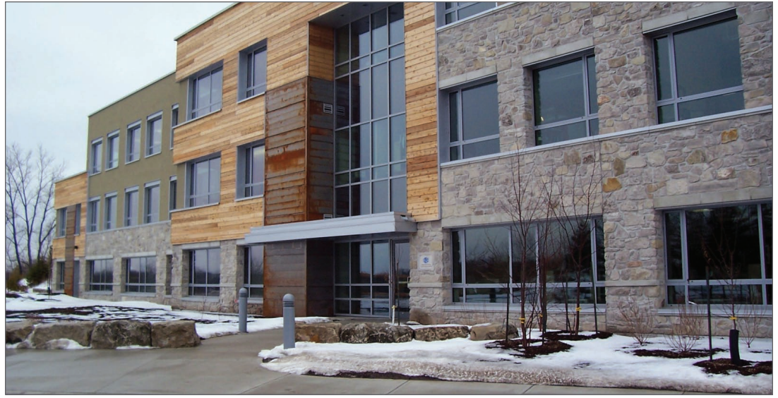
PHOTO CREDIT ENERMODAL ENGINEERING
