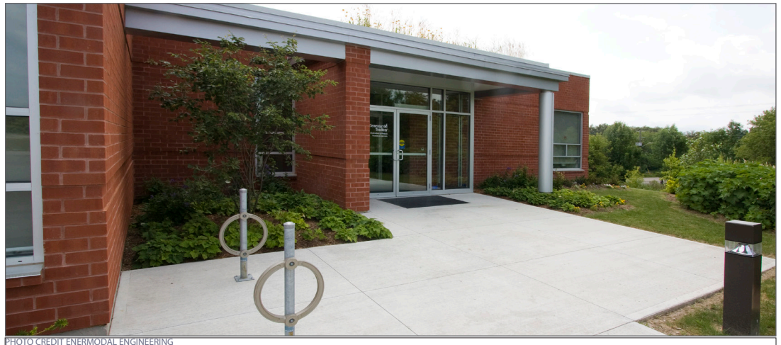
PHOTO CREDIT ENERMODAL ENGINEERING
