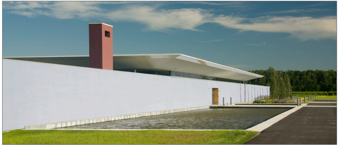
PHOTO CREDIT ENERMODAL ENGINEERING
