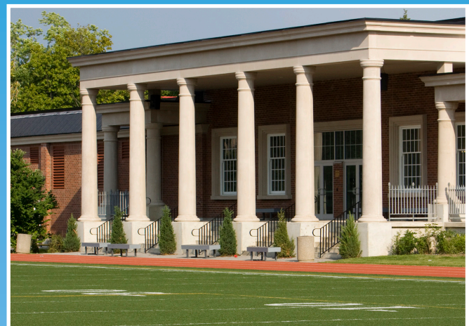
William P. Wilder '40 Arena & Sports Complex, Upper Canada College (Toronto, Ontario) LEED Gold certified
