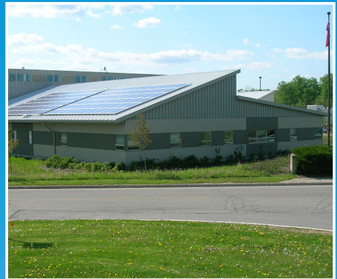
Waterloo Region EMS (Cambridge, Ontario); LEED Gold certified
