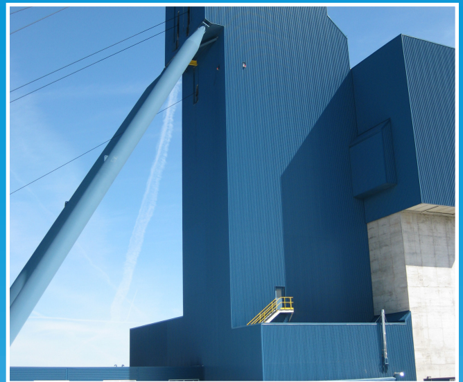
Xstrata Nickel Office and Dry Complex (Sudbury, Ontario) LEED Gold certified
