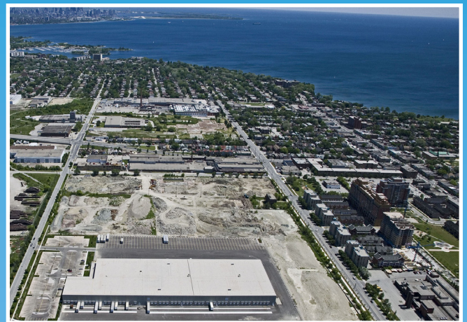
Canpar Distribution Centre (Toronto, Ontario) LEED certified
